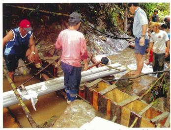
Constructing dam for gravity-feed water supply at Long Sabai
